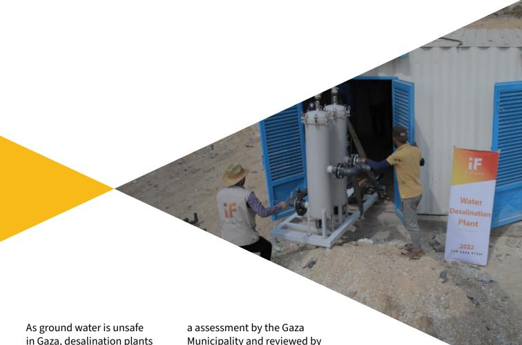
As ground water is unsafe in Gaza, desalination plants provide a crucial lifeline to local communities and their access to safe drinkable water. The Tal Al-Hawa water desalination plant was not functioning to specification. The plant's technical specifications were insufficient for the water characteristics of local area. This was confirmed through
